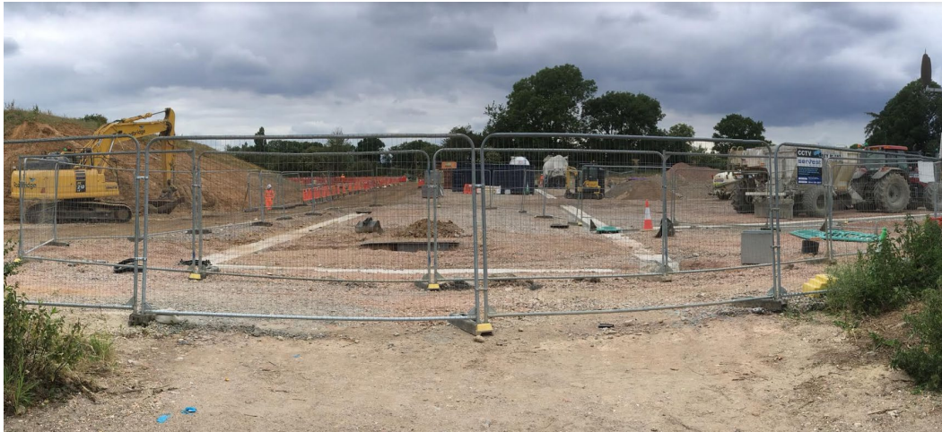
Figure 2: HS2 works near Denham
