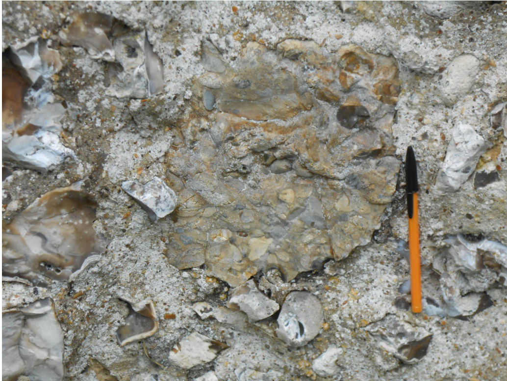
Figure 6: A block of Buckinghamshire Puddingstone in the church wall at Bradenham Manor.
